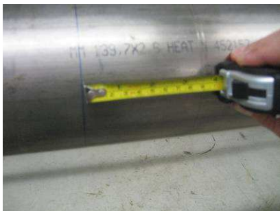
Picture 29 Measure required distance (given by flow transmitter)
