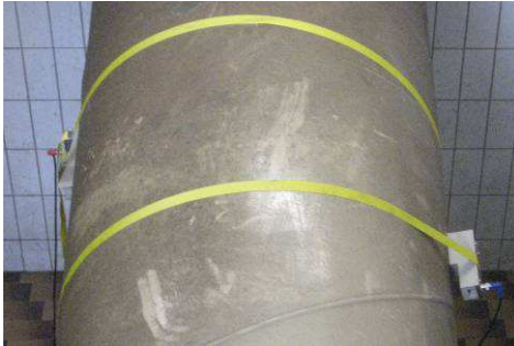
Picture 21 Example of Z-mode installation with fabric-reinforced tensioning tapes for large pipe diameters
