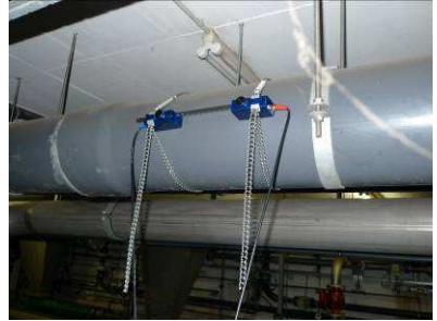
Picture 11 Preferable mounting positions for ultrasonic transducers (2)
